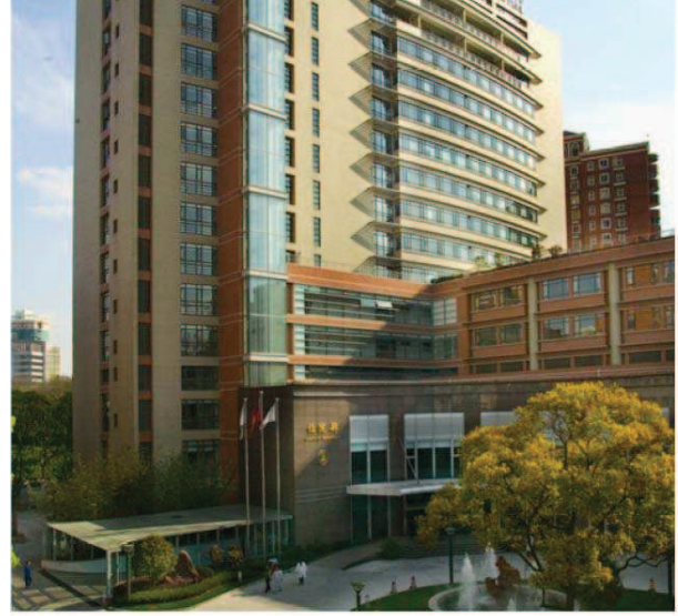
Figure 9 : The new Shanghai Chest Hospital, Shanghai, China--2006
